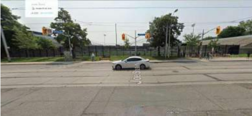
Street view on King Street West facing the North side of the Stadium on Google Maps .
